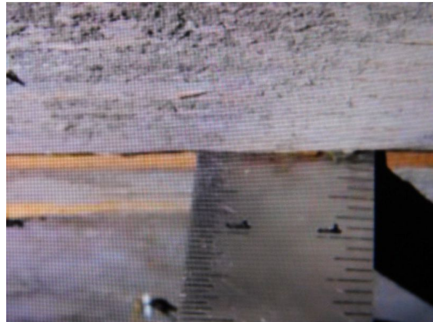
1/2" Deck Thickness Confirmed
