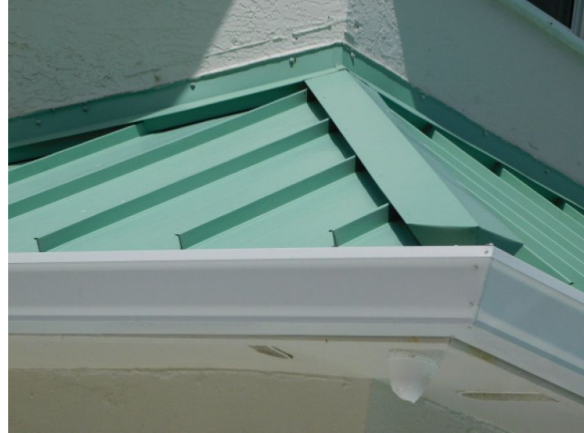
Metal Roof Covering
