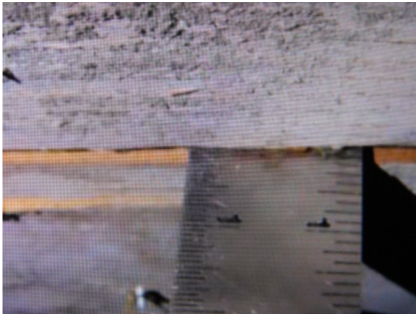
1/2" Deck Thickness Confirmed
